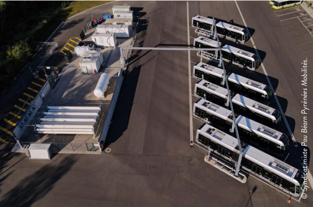
▶ Figure 7: HRS with on-site hydrogen generation in Pau, France. An H2 production and storage facility is shown at the left of photo. Buses are sequentially refueled overnight at their parking bays. The high level of redundancy in terms of dispensers at this site is exceptional.
