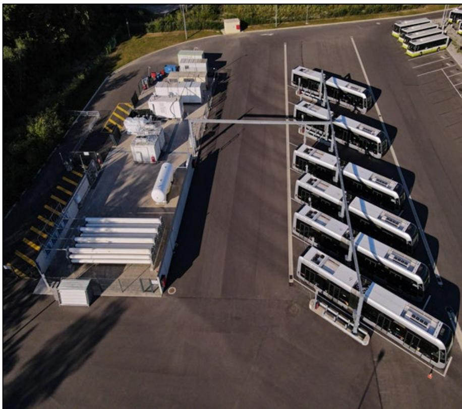
**Figure 4-4: HRS with on-site hydrogen generation in Pau, France.** H<sub>2</sub> production and storage facility is shown at the left of photo. Buses are sequentially refueled overnight at their parking bays. Photo by permission of Syndicat mixte Pau Béarn Pyrénées Mobilités.
